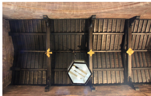
The inner south aisle has shallow king-post trusses. The roof to the outer south aisle is replaced
